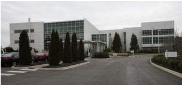
The Rawlings Group building in La Grange is on Eden Parkway. (By Pam Spaulding, The Louisville Courier-Journal) December 8, 2009
